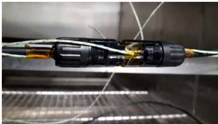
Figure 1. Thermocouple mounted on DC connector surface
